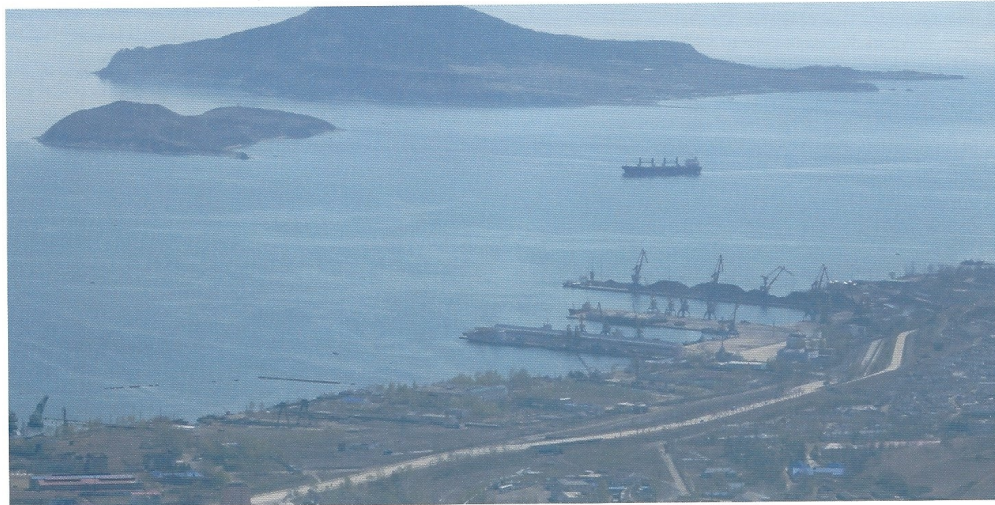
The harbor of Rason: the right-hand pier is rented to Russia; in this photo of 2016 coal can be seen; currently the Russian pier is empty, while small amounts of coal are shipped from the middle (North Korean) pier.
